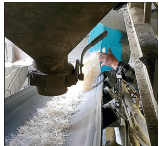
SafeTcrete™ Fiber added to mixing conveyor at casting site.
